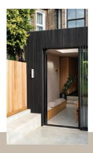
The interior was clad with ThermoWood Iroko, our offering natural and complimenting the Tsubo within the home. Both our natural ThermoWoods and ThermoChar® materials offer 30+ years of durability, are extremely stable and resistance to rotting, warping and cupping, making them a great choice for internal and external use.
